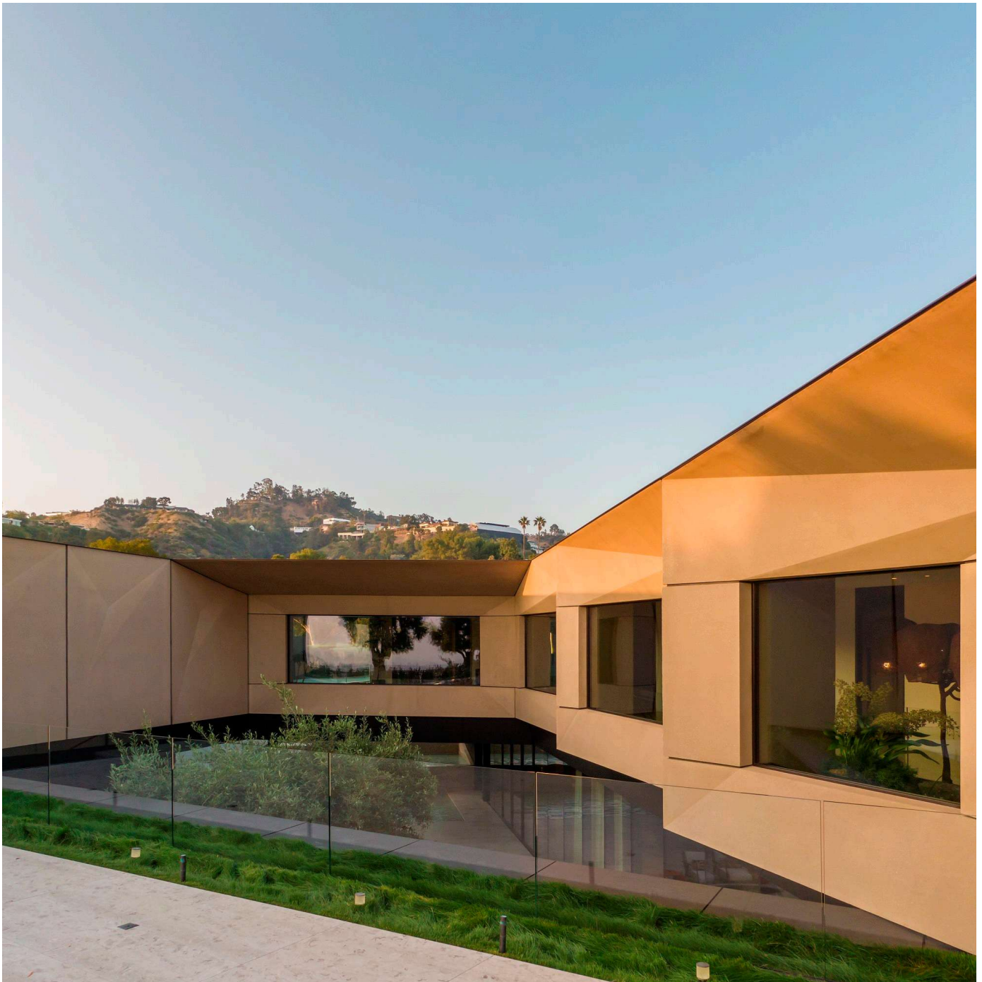
Glass-reinforced polymer panels make up the facade (Fernando Guerra)
